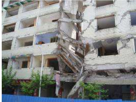
Aftermath of the 2008 Sichuan earthquake. 7
